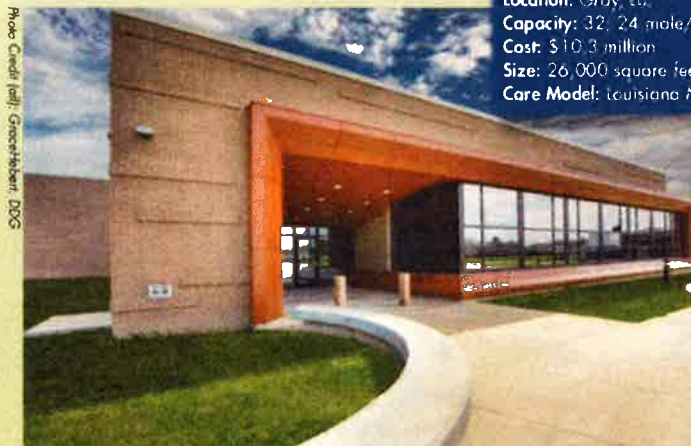
The building should age well thanks to the county's request that GraceHebert and DDG design it to meet Category 4 Hurricane Standards.
