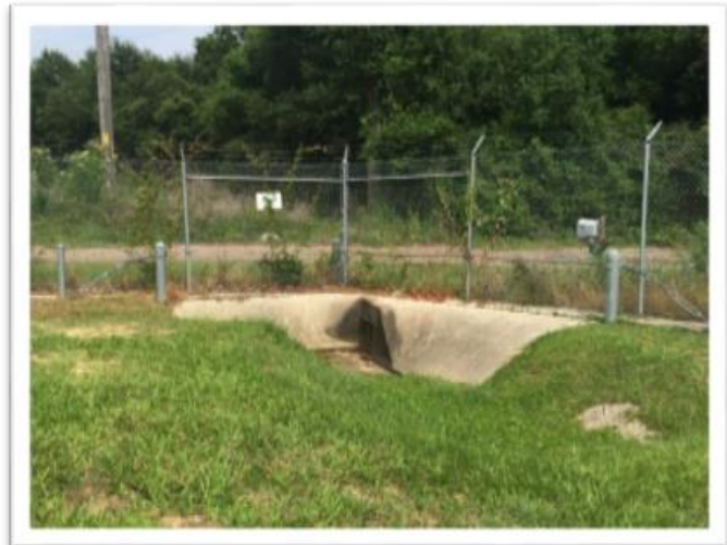
Figure 53 Drainage canal located within NCBC Gulfport
