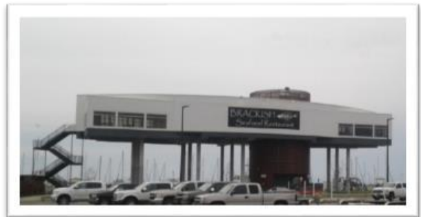
Figure 15 New construction in Gulfport (above) and Long Beach (below) depicting the additional construction standards after Hurricane Katrina
