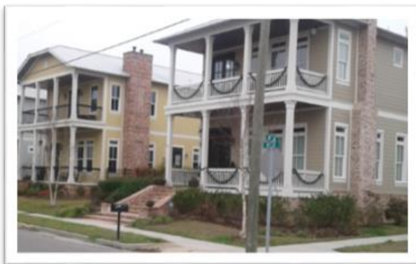
Figure 13 Recently constructed houses off of Highway 90 in Gulfport
