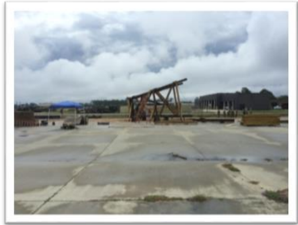
Figure 25 Construction training exercises
