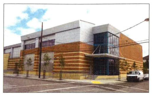
block with reinforced cells at 16" O.C. The CMU block wall system will resist the harsh chemical that are required to regulate the natatorium pool water.
