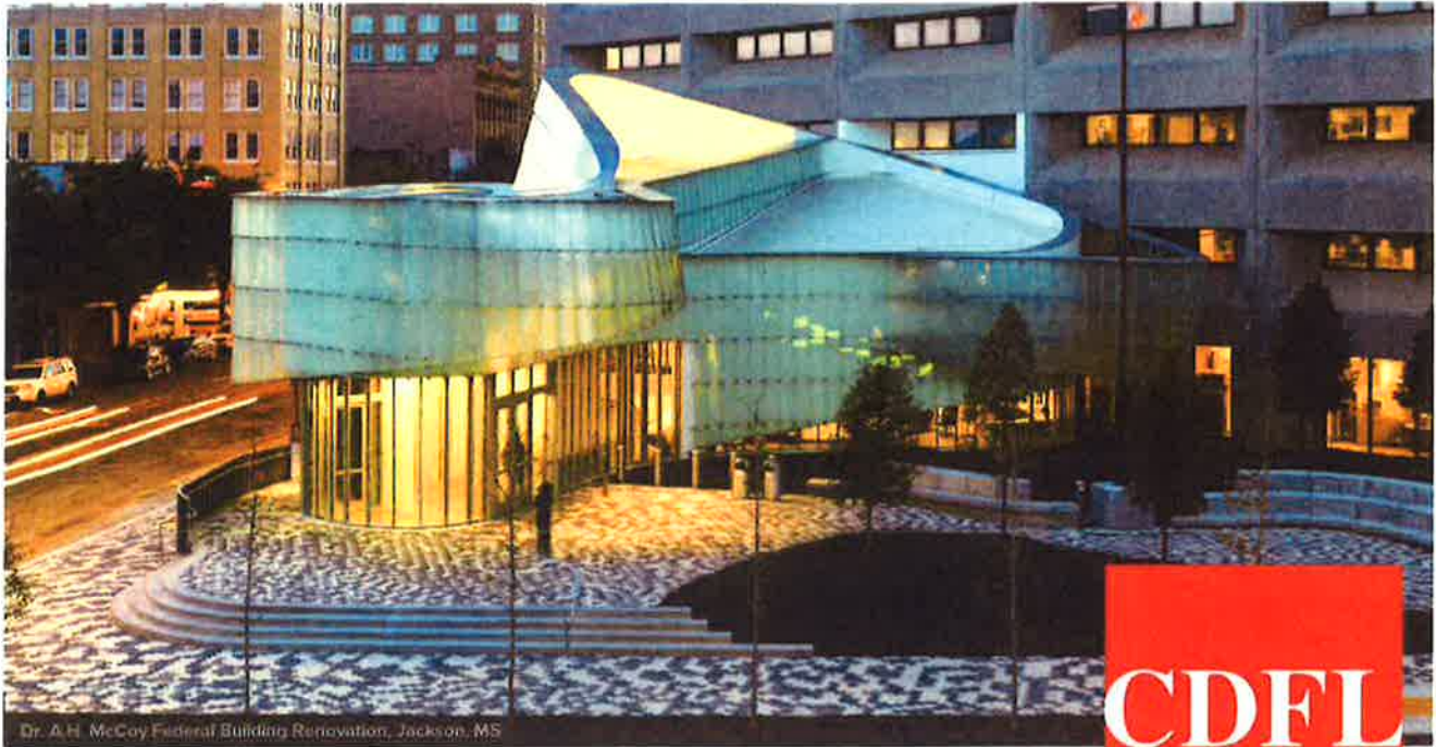
Dr. A.H. McCoy Federal Building Renovation, Jackson, MS
