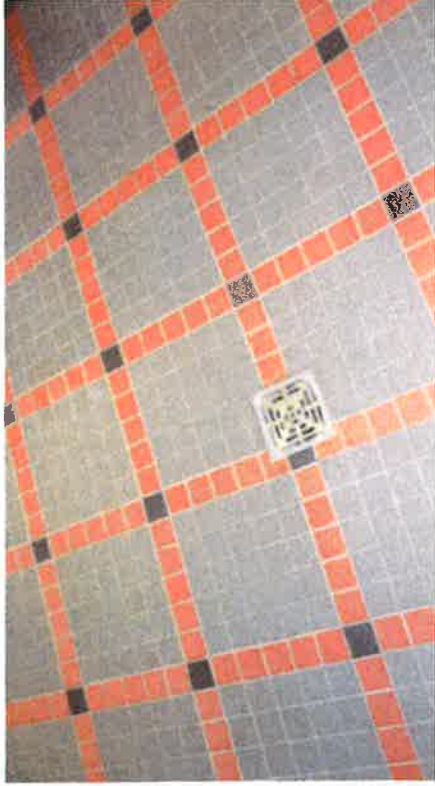
New Tile Floor in Field House Renovation
