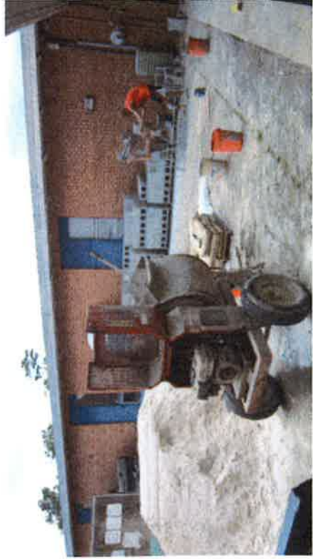
Contractor Work Area
