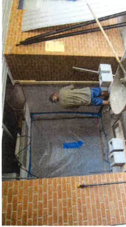
Concrete Masonry Work - Before
