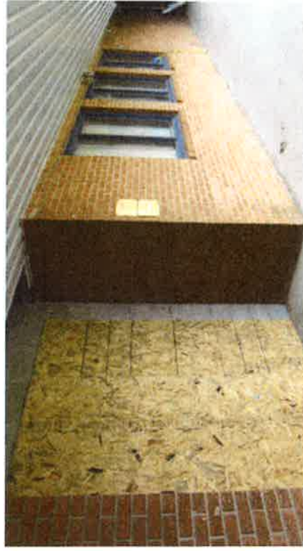
Concrete Masonry Work - After
