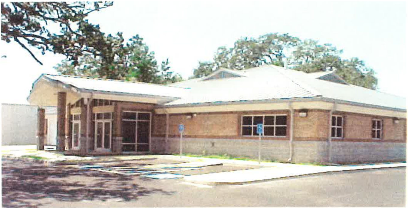
Harrison County Department Human Services Building – Biloxi, MS
