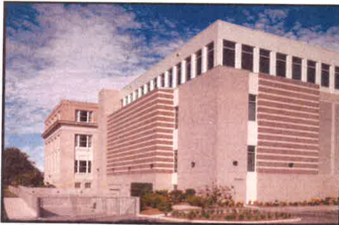
Highlands County Courthouse & Jail Sebring, Florida
