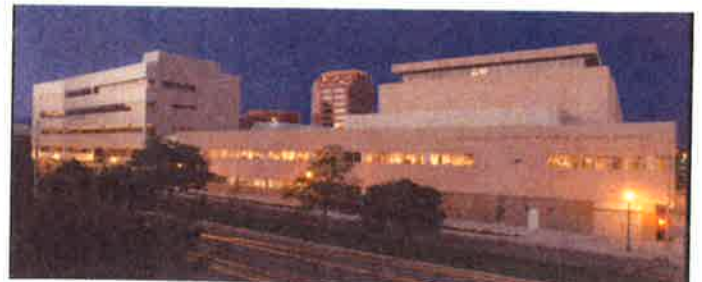
El Paso County Courthouse Colorado Springs, Colorado 189,000 SF Addition
